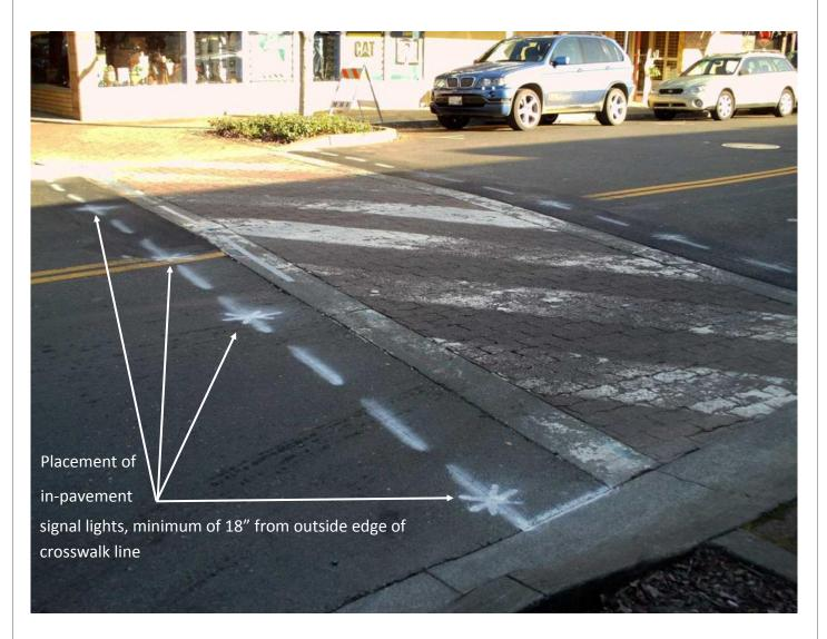
Below is a typical mid-block crosswalk with 7 in-pavement signal lights on each side. The "Zone of Convergence" is the area in the traffic lanes where the signal light lenses are aimed towards <u>approaching motorist</u>. The signal lights will merge at the eye level of the approaching driver. This "Zone" is typically located 200 - 400 feet from the crosswalk zone (See Installation Manual Section 3.7)
