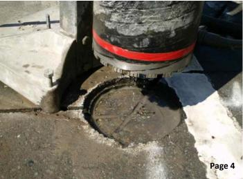
Install all necessary wire to predetermined connection points and lay in cleared roadway cuts. (See Installation Manual Section 3.6). Place material on top of the wires into the saw cut at the core drill entrance area to hold down the wires & simultaneously plug (see picture to right) the core drill area to prevent flow of epoxy back into the saw cut.
